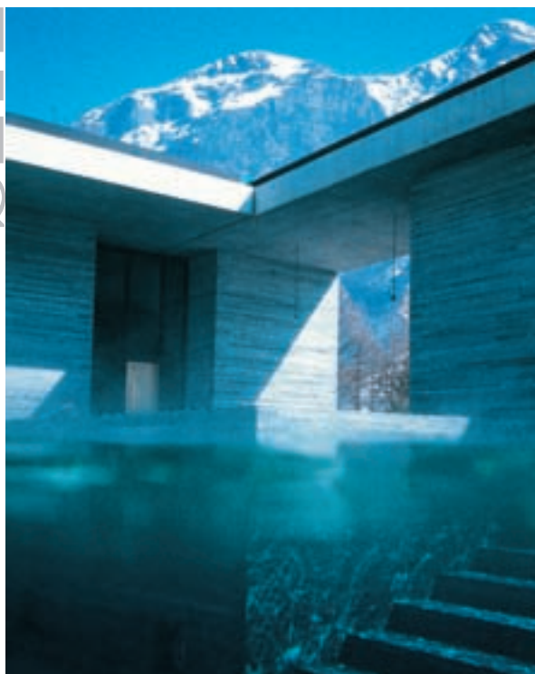
Vals: The rectangular building comprises 60,000 superimposed slabs.
